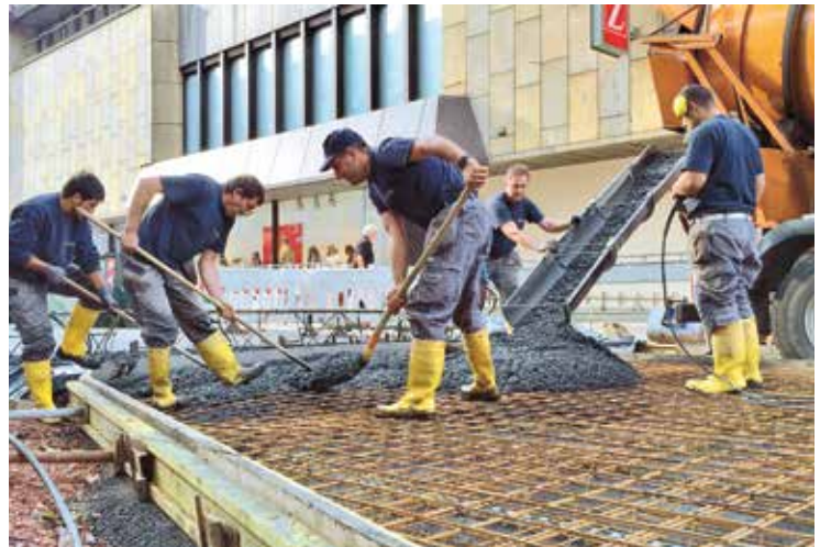
Abb. 9: Betonage
